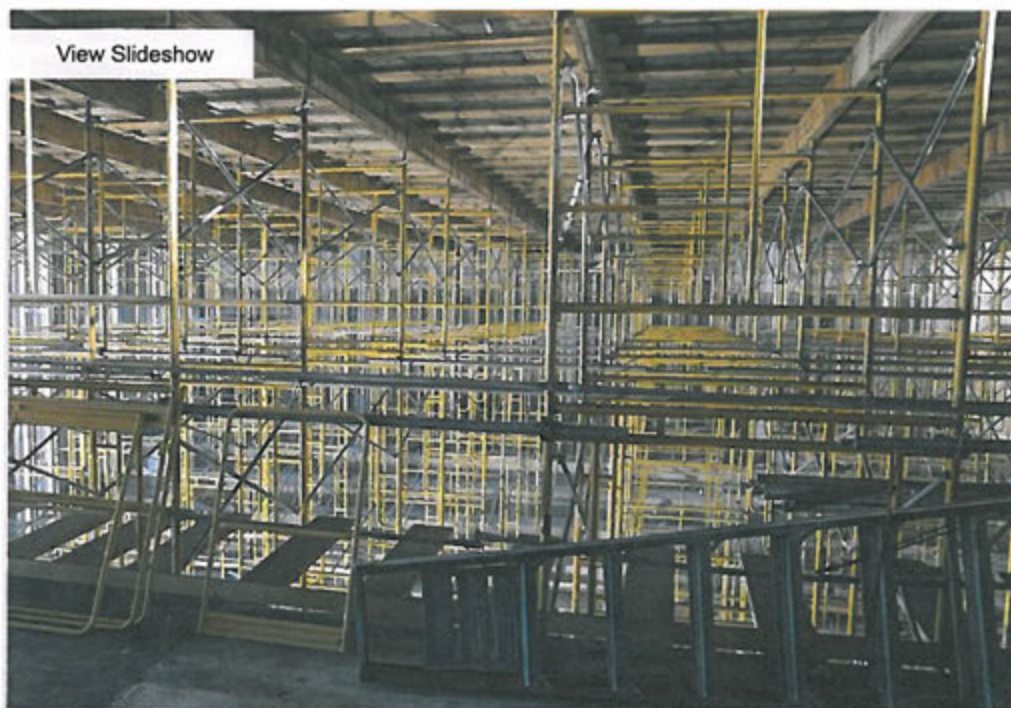
Scaffolding in the concert hall as work continues on the Voxman Music Building in Iowa City on Monday, Nov. 2, 2015. (Stephen Mally/The Gazette)
